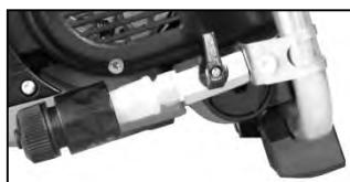
water supply closed (valve lever across)
